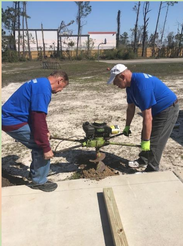
Two man auger for our fence posts at the Shelter
